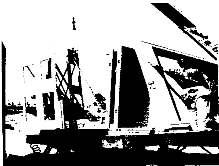
Load bearing shear panels to 40 ft. high.
