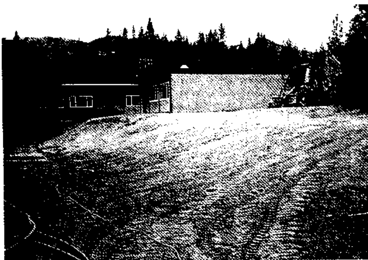
Back yard of Trinity High School in the area of loop installation which has been graded pending reseeded
