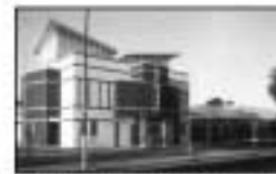
West Contra Costa USD Bond Program, $450 Million Program and Construction Management
